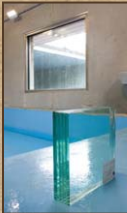
It took five layers of sturdy glass laminated with plastic to create the viewing window (left) into the hippo quarters. Space in the outdoor giraffe yard was expanded by using a fence with horizontal cables instead of a full moat. Skylights provide natural light for the giraffe indoor exhibit.
