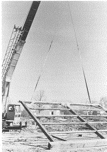
Construction officially began with the raising of the wall.
