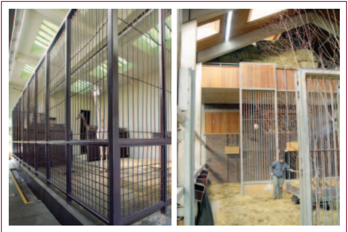
Beautiful wood surfaces frame large giraffe stalls at the Cologne Zoo (right). Giraffe stalls at the Milwaukee County Zoo (left) will be revamped completely, using some of features from Cologne. Photos of European zoos are by Bruce Beehler.
