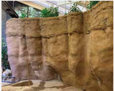
Contractors added three feet to the wall.
